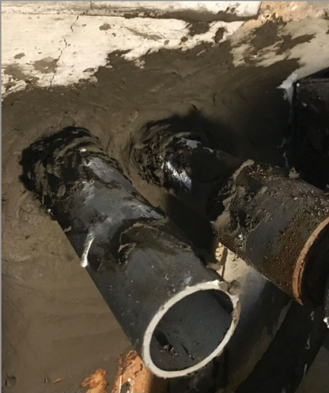
Step 4: Cover foam with a thin layer of concrete thin-set
